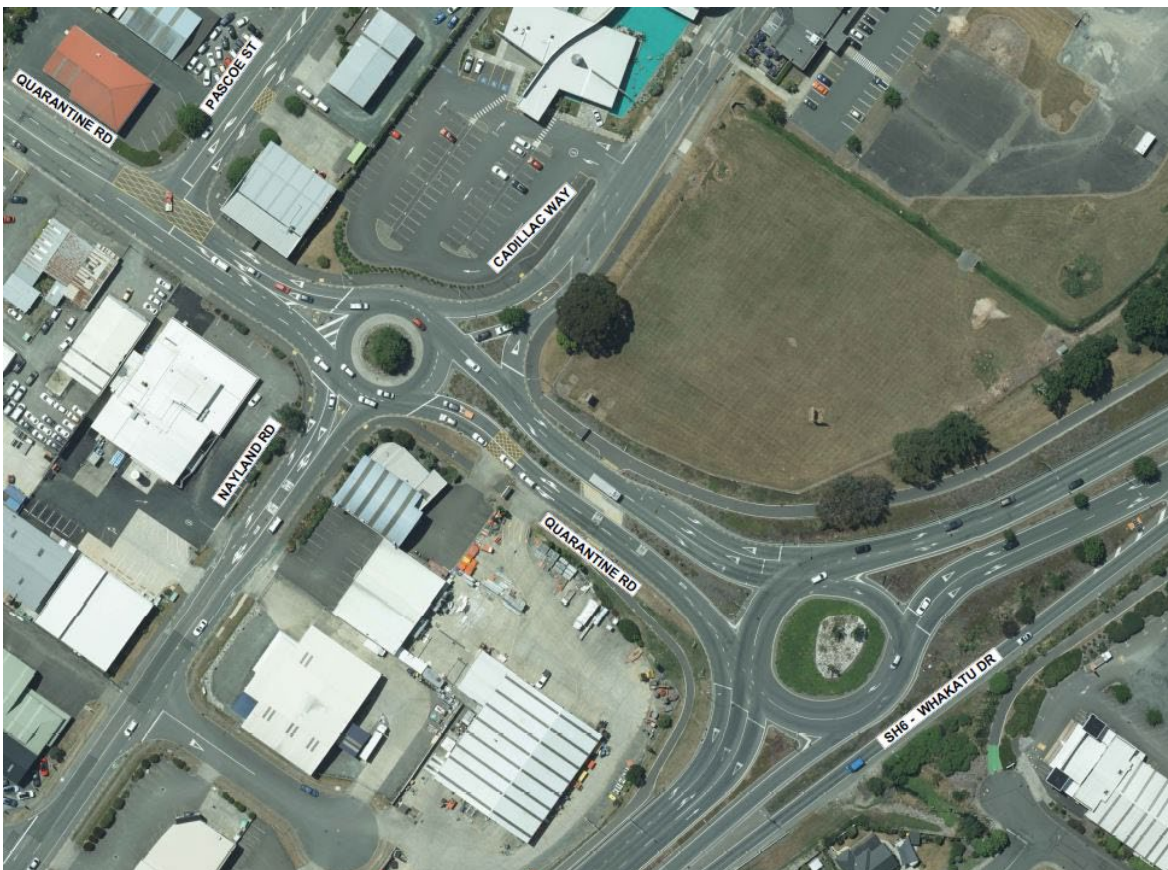
Figure 3-3: Quarantine Road Intersections
